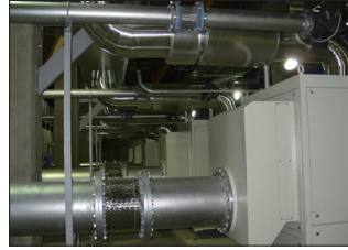
WWTP of Suji, Youngin(NX300), Korea
